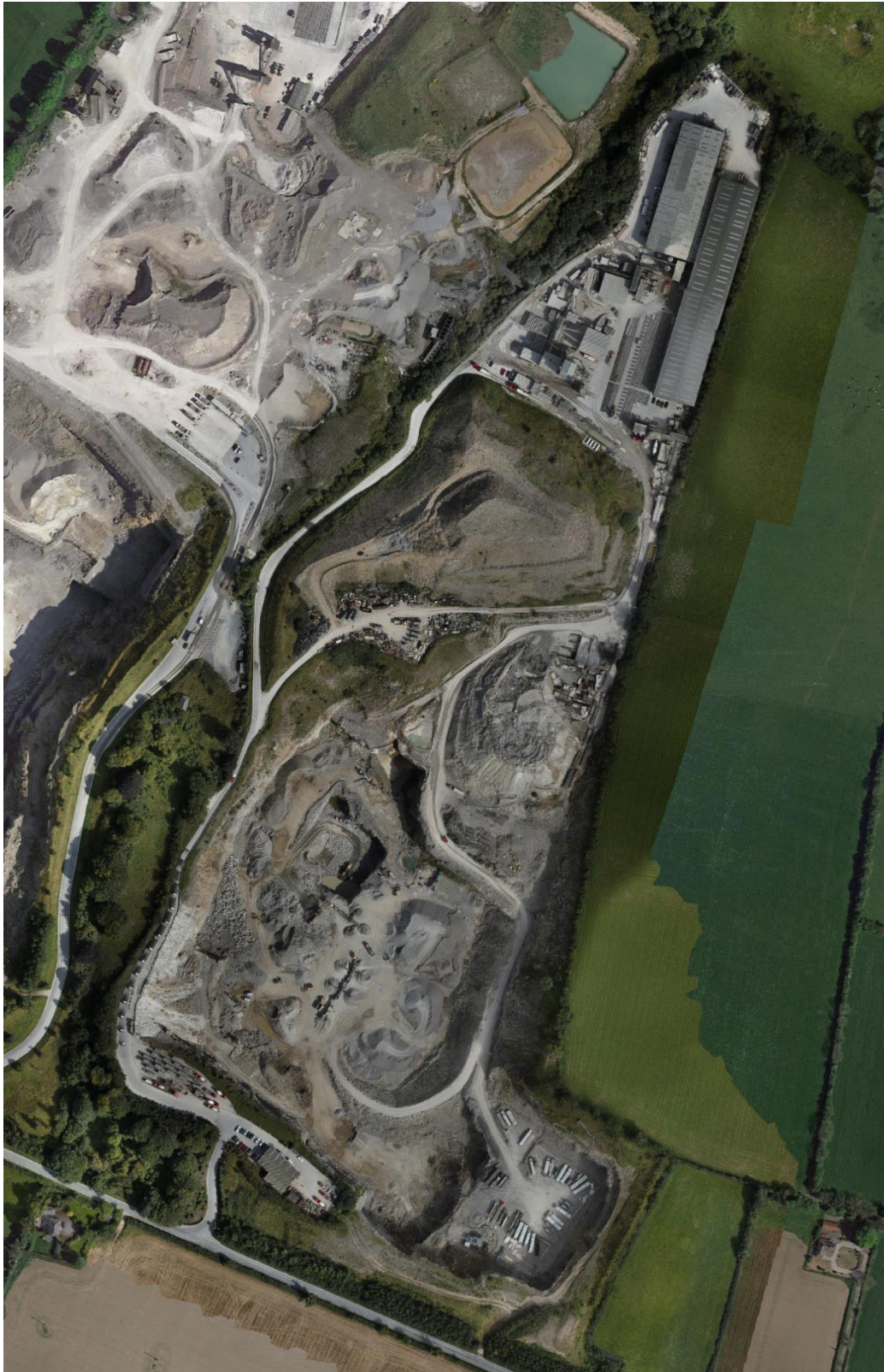
Figure 3.1 – Orthophotograph of Site- 17 August 2023
